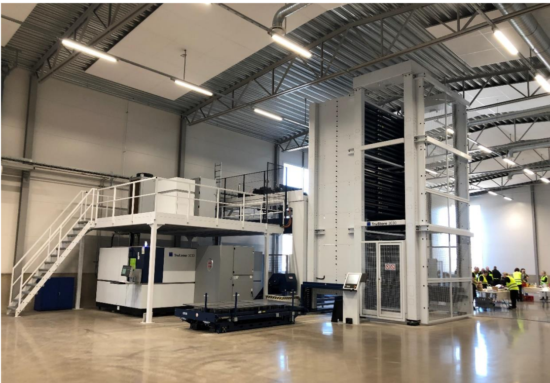
The fiber laser unit is the centerpiece in the new factory building.
